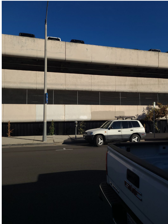
Northeast of site ○
