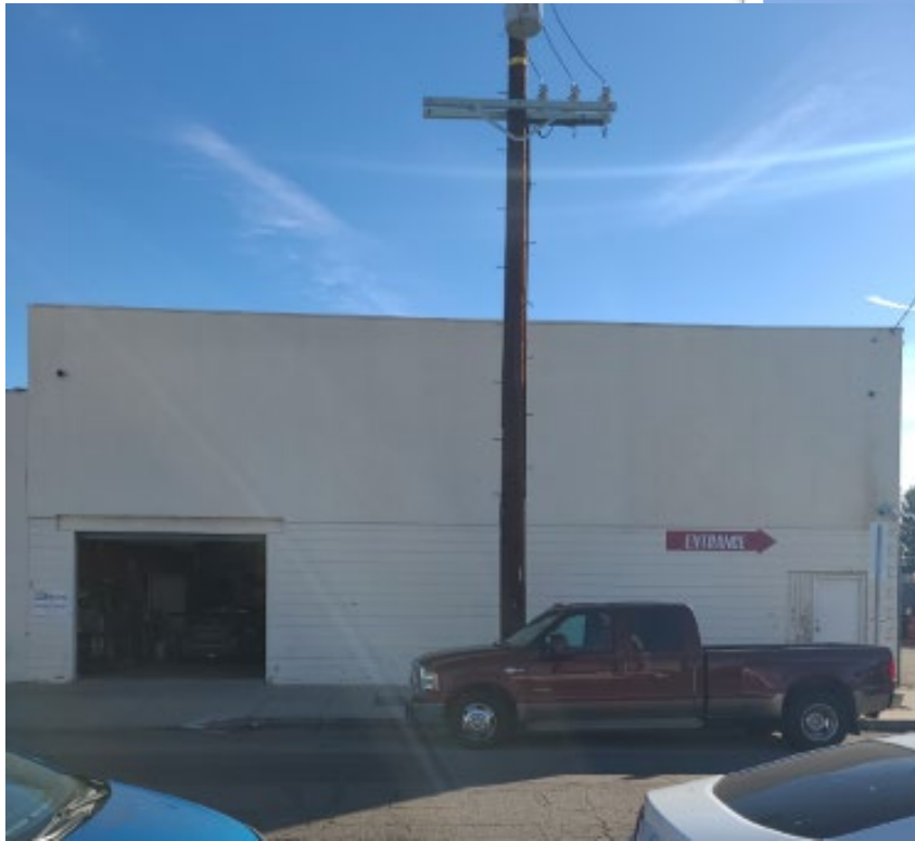
East façade rollup No. 2 and customer entrance
