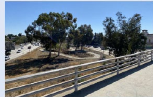
Before: Vermont Ave Overpass.
