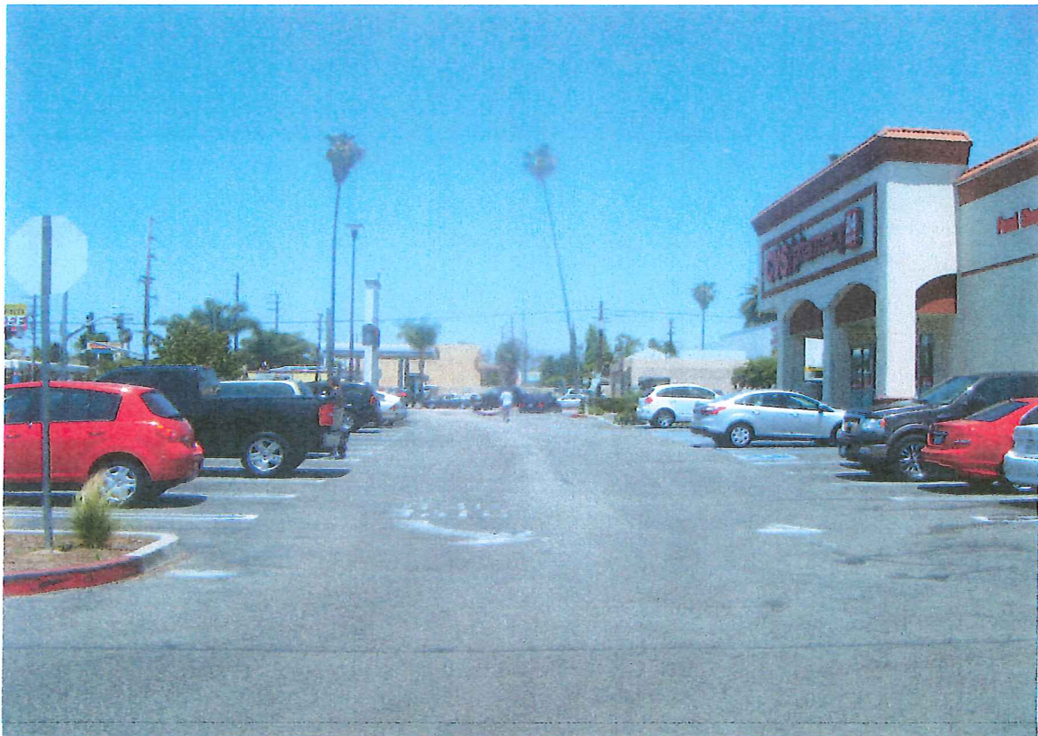
14. 15232 Sherman Way: view looking north at the parking lot on the west side of the building.
