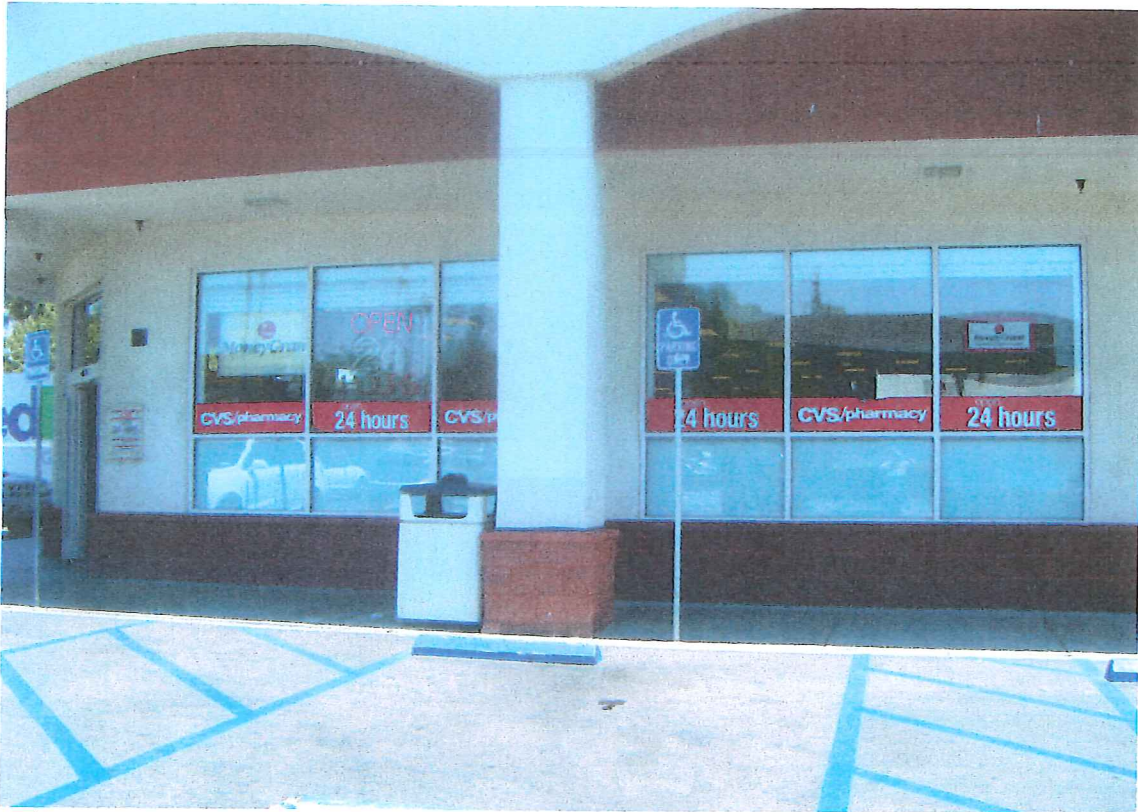
5. 15232 Sherman Way: view looking at the windows on the west side of the building.
