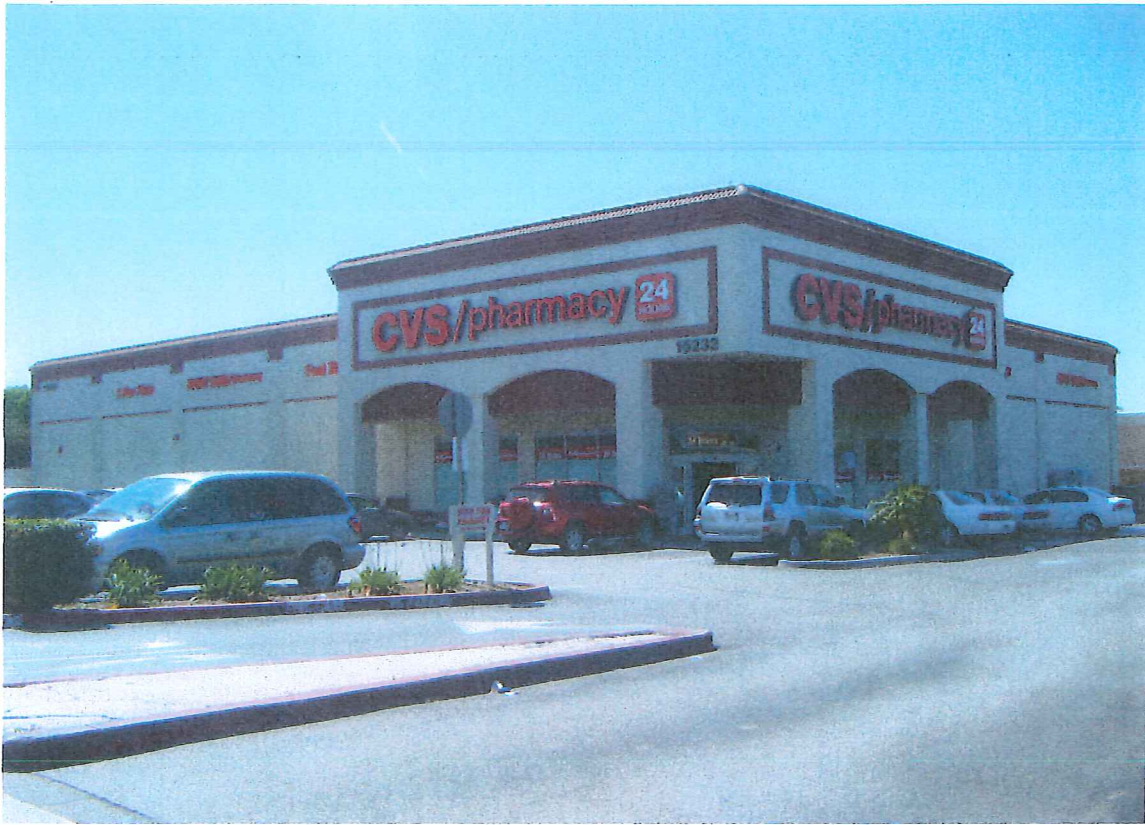
1. 15232 Sherman Way: view looking southeast at the front entrance of the subject property.
