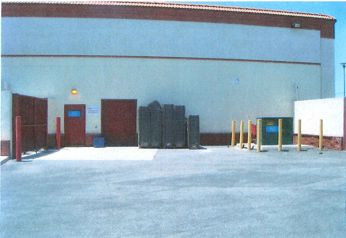
10. 15232 Sherman Way: view looking west at the loading area on on the east side of the building.
