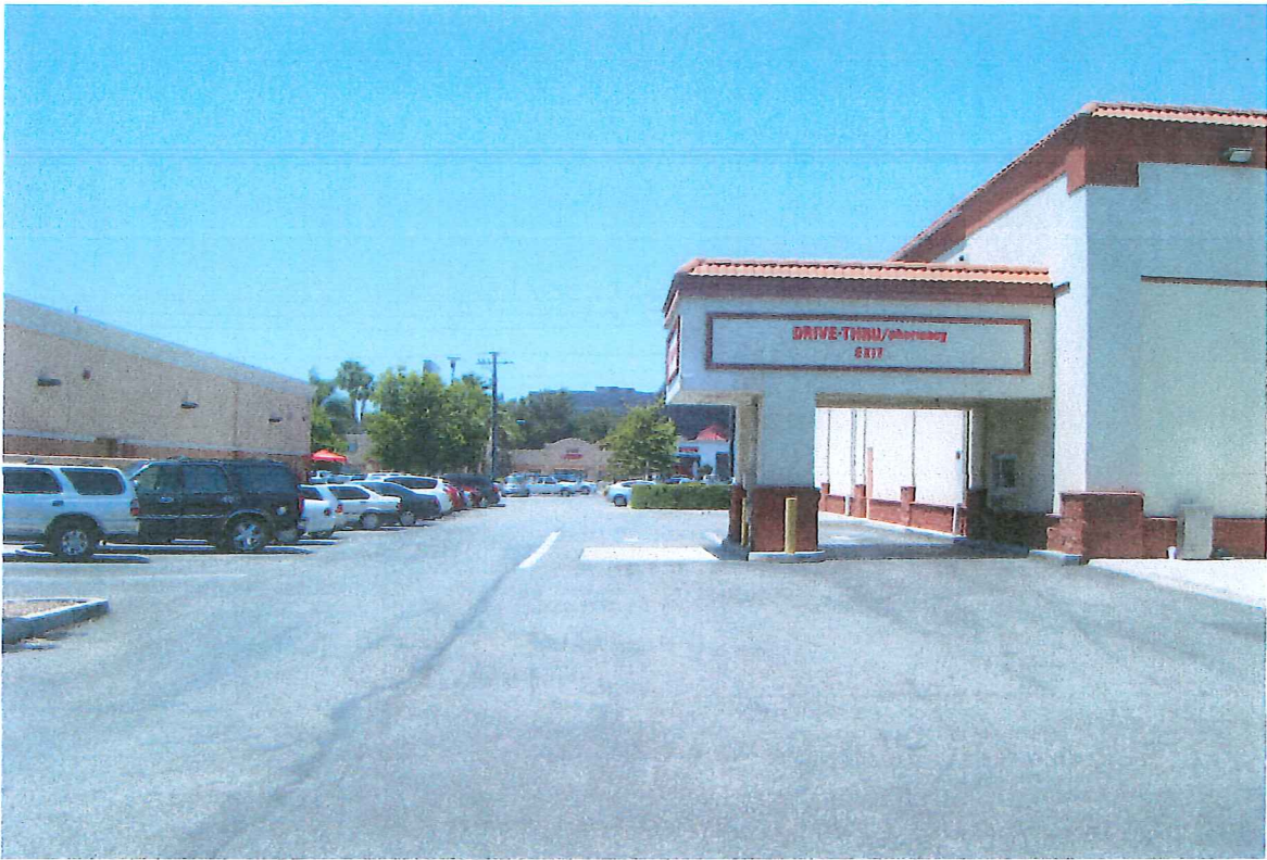
9. 15232 Sherman Way: view looking west at the Pharmacy window on the south of the building.
