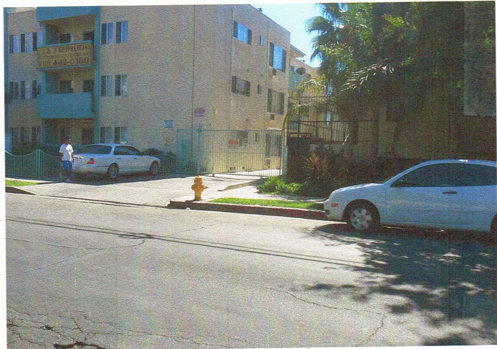
SOUTH - 14401 VALERO ST.
